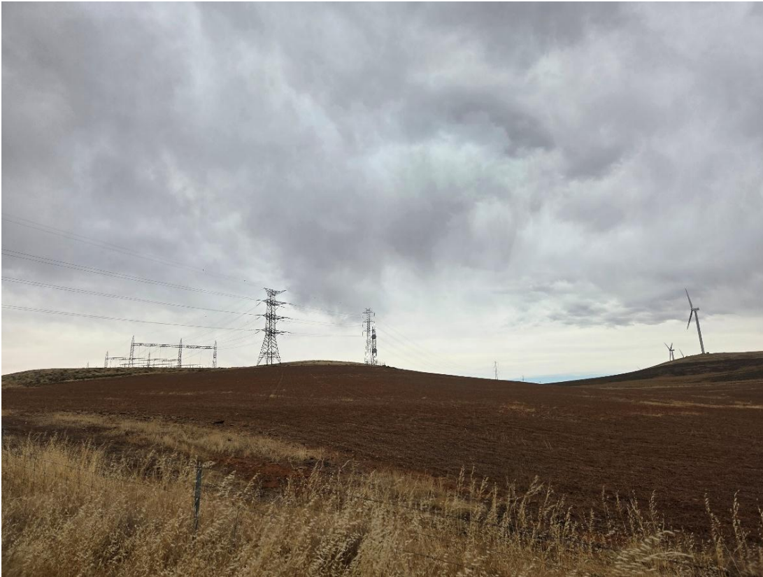
Photo 4.1 Western side of the Belalie Substation Expansion Area. View looking south-east toward existing Belalie Substation from Gilfillan Road. WTGs from the Hallet Wind Farm shown to the right
