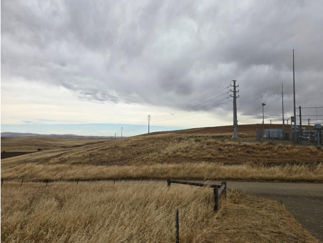
Photo 4.2 Eastern side of Belalie Substation Expansion Area and western end of the OTL Area. View looking south from Gilfillan Road, with the existing Belalie Substation shown on the right
