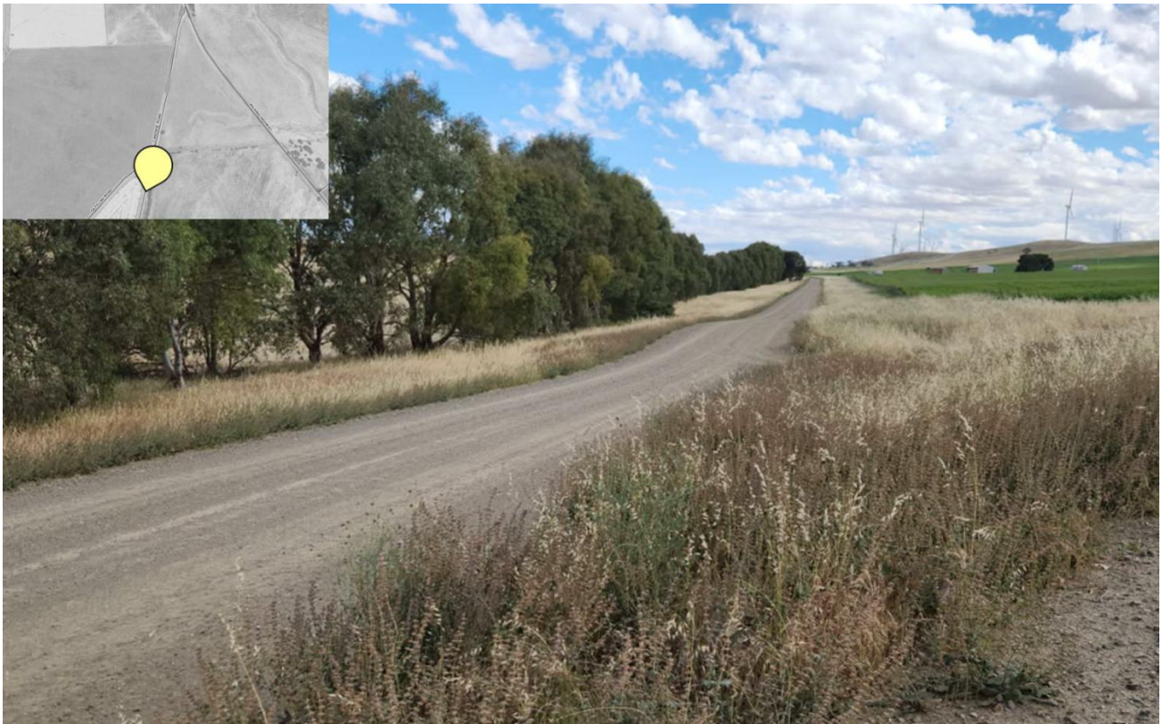
Figure 6.10 Canowie Road (Empirical Traffic Advisory Pty Ltd, 2026)
