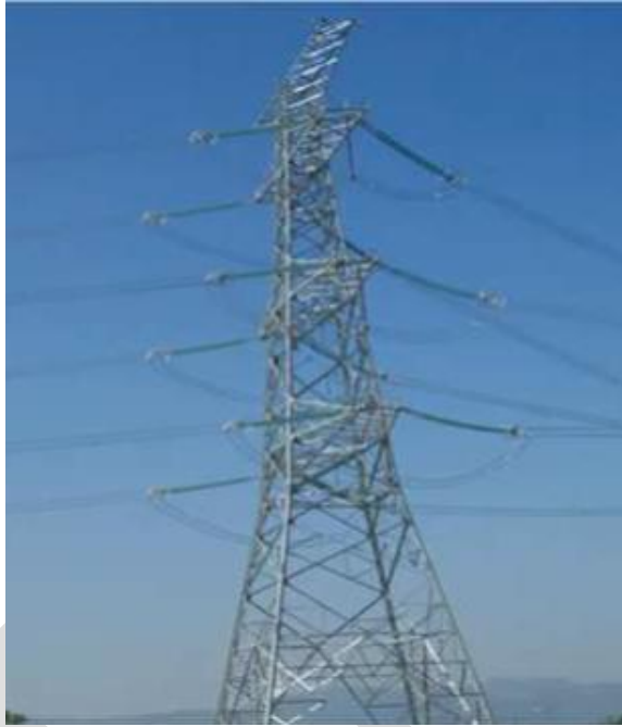
Photo 4.20 Example of a typical 275 kV OTL tower (Wax Design, 2026)
