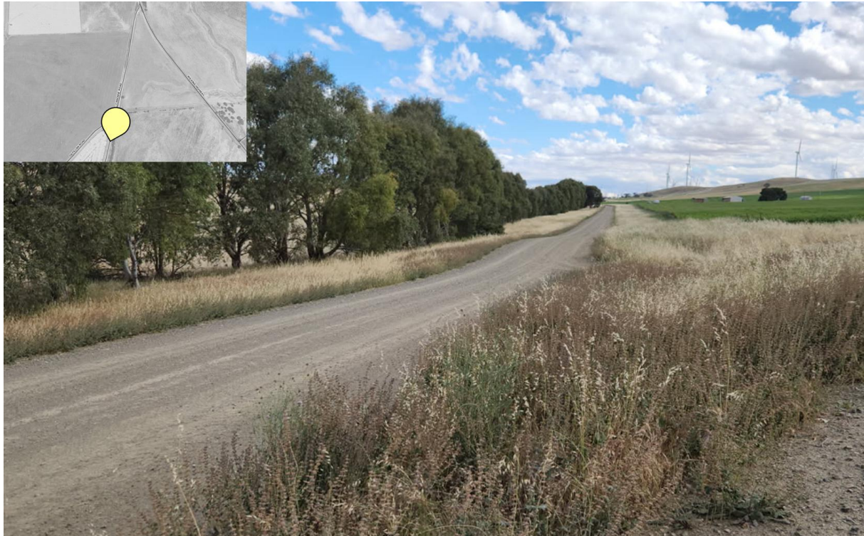
Figure 5.3: Canowie Road / Gilfillan Road Intersection - Looking South
