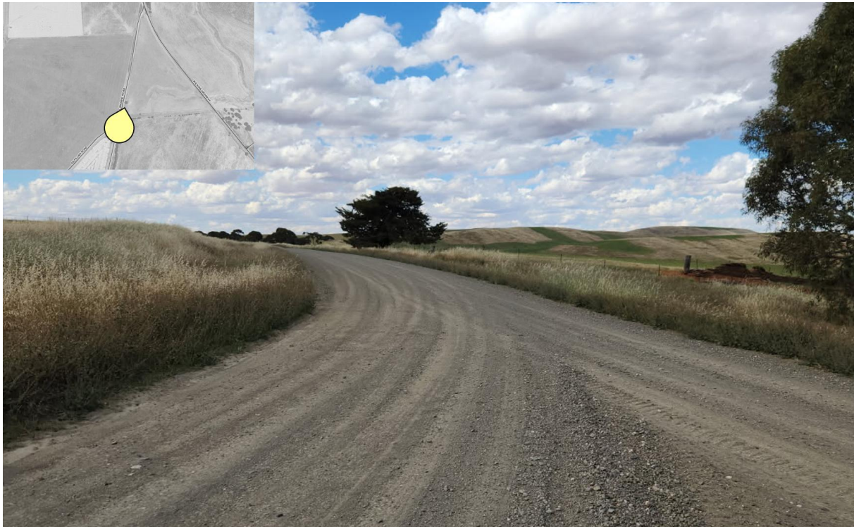
Figure 5.4: Canowie Road / Gilfillan Road Intersection - Looking North
