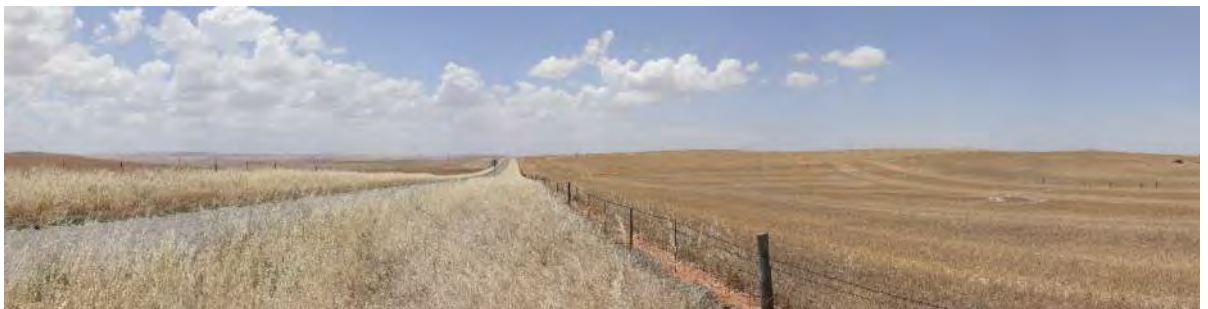
Figure 23: Digital Overlay showing the transmission line lattice towers: Viewpoint 3
